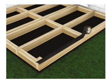
The maximum recommended space between 3-111 space between Joist rows depends on the angle at which you intend to lay your boards in relation to the Joists, but should never exceed **40cm**, please see diagram. Apply Deck Tape to the top surface and cut ends of the timber joists to protect them from moisture.
